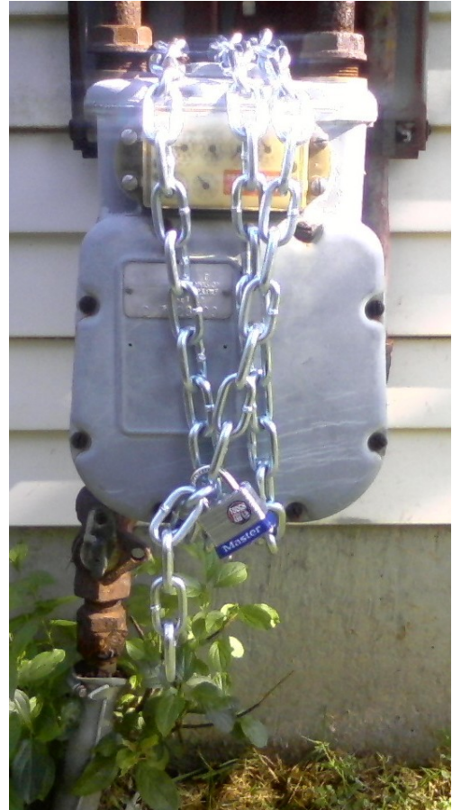
Gas meter. Note the meter at the top. Note the chain wrapped around three times and secured with a lock through two loops.
