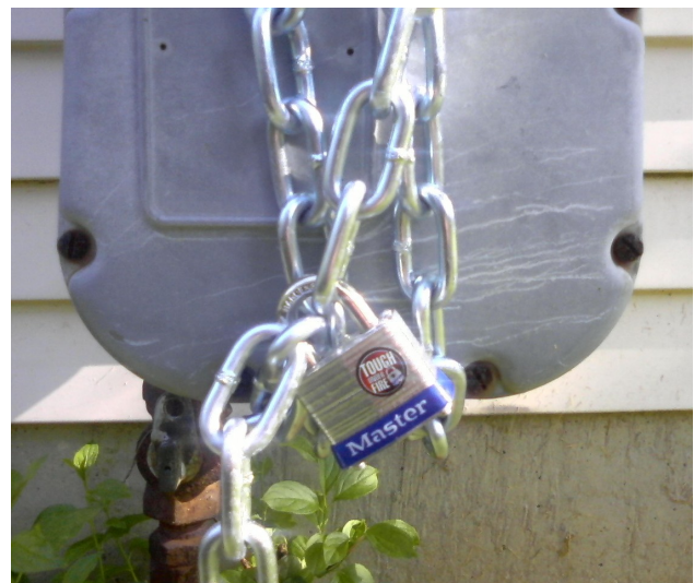
Close-up of lock on gas meter.
